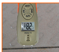
Trace water leakage on walls, floors, ceiling, carpet
