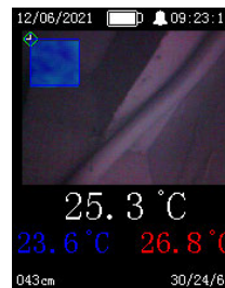
Auto trace water leaks, under ceiling; walls; ground floor; basement.
